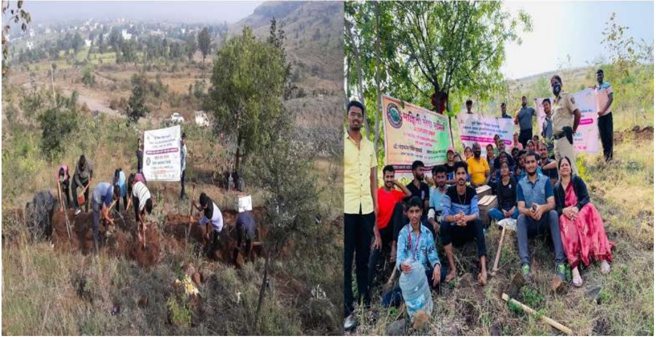
Work for the purpose of water conservation and water horizontally by digging continuous counter trenches(CCT) on the Bakori hills.
